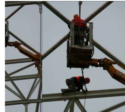
2 Alternative: Accessing the truss via a cherry picker
