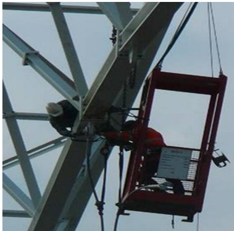
3 Team work for complex steel construction assembly
